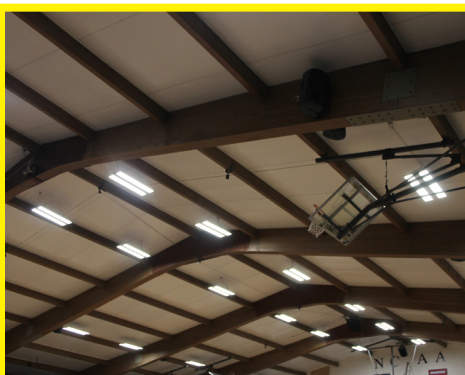
In addition, the ceiling mounted volleyball standards were removed and each Glulam wood beam had metal support plates installed to reinforce small cracks they had substained.
