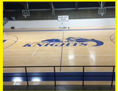
Part of the Summer Improvements included the refinishing of the gymnasium floor. The playing surface was sanded down, repainted with a large Knight logo at midcourt and then refinished.
