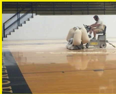
Part of the Summer Improvements included the refinishing of the gymnasium floor. The playing surface was sanded down, repainted with a large Knight logo at midcourt and then refinished.
