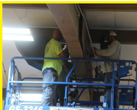
In addition, the ceiling mounted volleyball standards were removed and each Glulam wood beam had metal support plates installed to reinforce small cracks they had substained.
